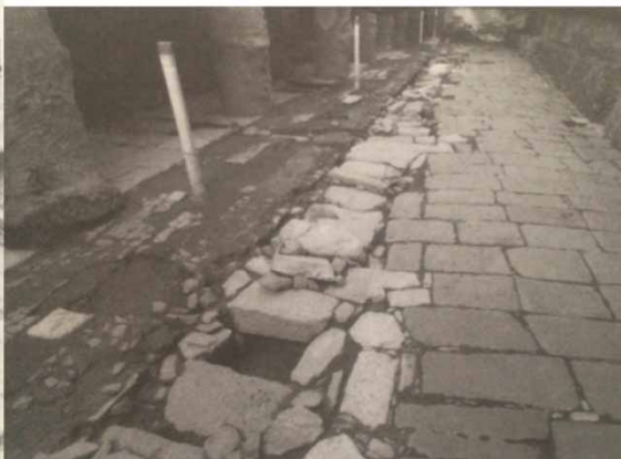
Figure 6 | Stone-built sewers of Byzantine times (6th c.) in Thessaloniki: (a) in Pastier road and (b) in Egnatia road.
