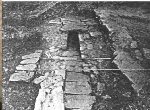
Figure 5 | Roman sewers; (a) central sewer covered with stone-built apsis in Thessaloniki and (b) on the island of Thassos (Antoniou et al. 2014).
