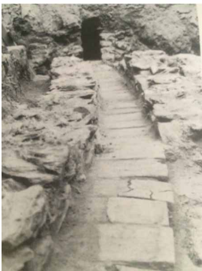
Figure 6 | Stone-built sewers of Byzantine times (6th c.) in Thessaloniki: (a) in Pastier road and (b) in Egnatia road.
